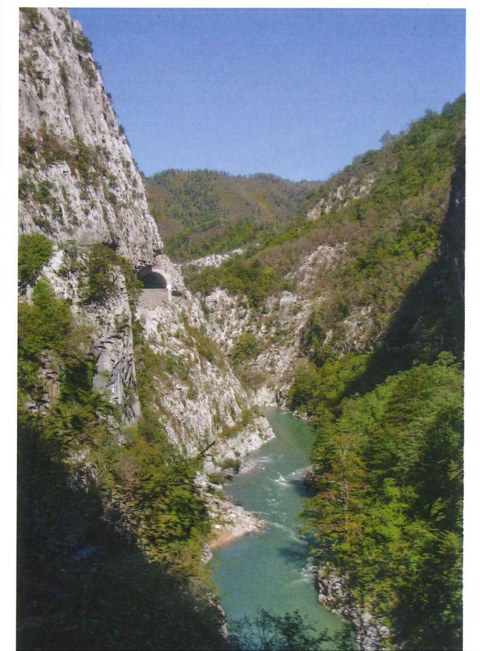
Source 1.22 Canyon of the Morača River in the Dinaric Mountains, Montenegro. A road tunnel has been constructed through the cliff on the left.
